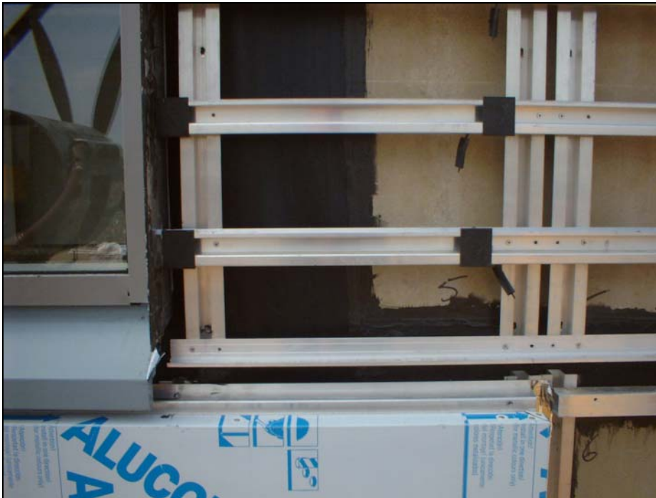
TERRACOTTA TILES REMOVED
