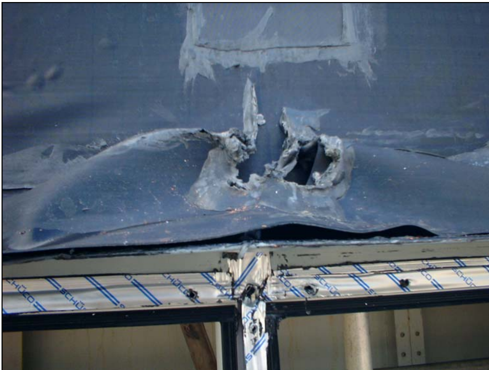
MENBRANE ABOVE CURTAIN WALLING
